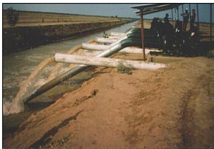
Irrigation scheme on the Senegal River
