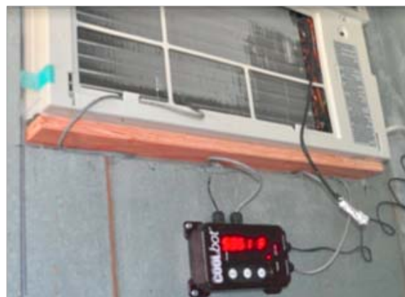
The Coolbot™ is a small black box that is wired into a standard air conditioner.
